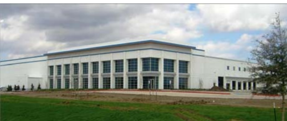
Republic Distribution Center – 312,522 SF
